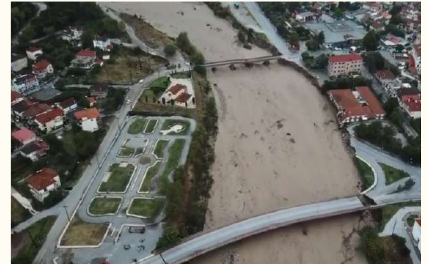
Damage from Ianos in Karditsa, Greece
